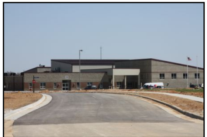
New Rogersville Elementary School
