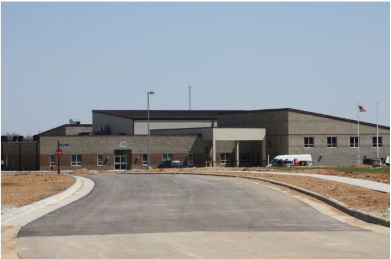
New Rogersville Elementary School
